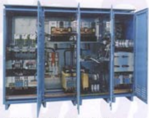
UPS 200 KVA for marine applications at Rina-LLoyd Register Standards
